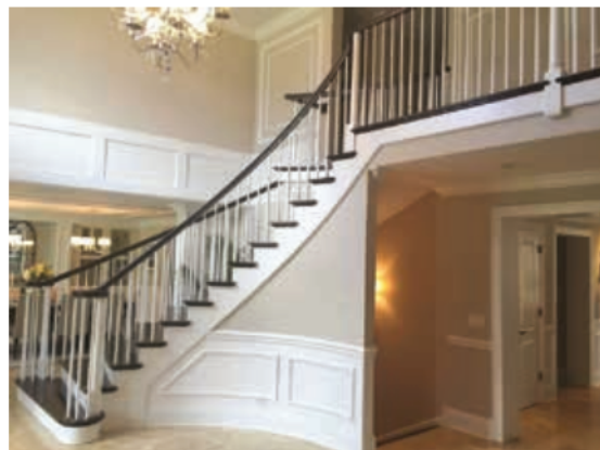
Foyer featuring two examples of wainscoting on the lower stairwell wall and lower portion of upper walls. Additional detailing lines the staircase while raised panel moldings form a dual box design on the upper front facing wall.
