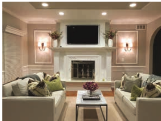
Picture framed sconces are just the tip of this well-planned trim and molding layout. Note the raised panel molding ceiling design further enriched by a white semi-gloss paint finish extending to the crown moldings.
